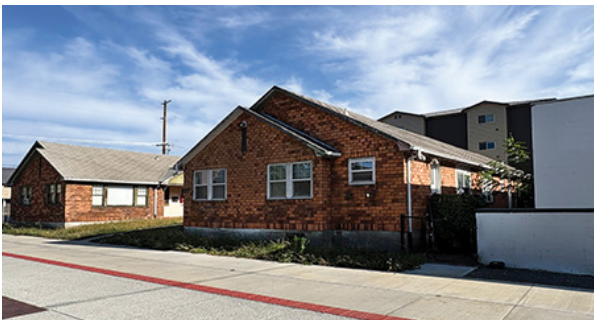
Property located at the corner of W. 13th St. and Jefferson across from the OHM Family Resource Center
