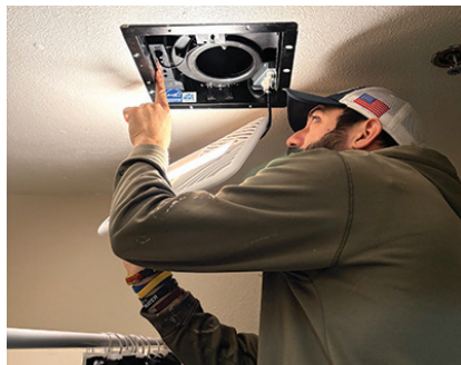
Installing moisture control exhaust fans
